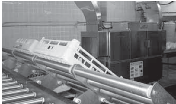
Norwood's new dishwasher with combined scraping table and soak sink.
