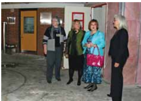
CEO Iris Neumann (right) tours one of the dining room construction sites with (from left) Administrator Betty Kolewaski, MLA Janice Sarich, and Culture Minister Heather Klimchuk.
