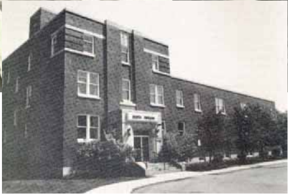
South Pavilion, also known as "The Annex" was built in 1947 (and torn down in 1995) and was Alberta's first publicly-owned long-term care centre and the place where our history began.
